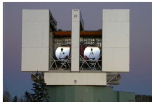
Figure 3: The Large Binocular Telescope on Mt. Graham, AZ combines light from two 8.4 m primary mirrors.
